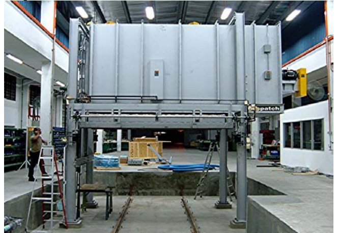
Figure 3: Doors hoisted and air plumbing completed. The very tight space for using lifting equipment and the pit made any placement of the heavy pieces a challenge.
