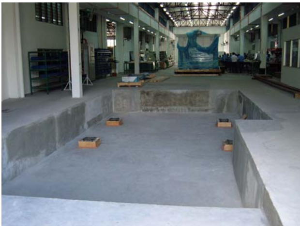
Figure 1: The start of the project. A concrete foundation consisting of a shallow pit is a part of the installation. The foundation was completed prior to the start of installation.
