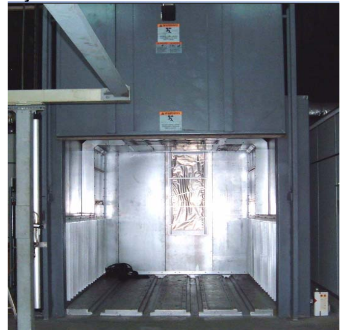
Figure 12. The door mast and door installed. The oven is mechanical complete.
