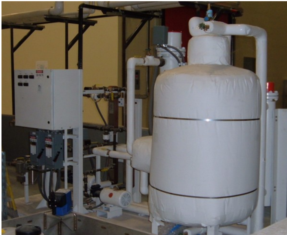
The picture shows the new heat separator installed at the customer site.
