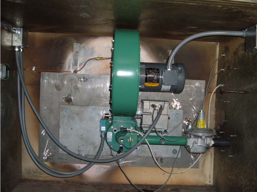
The new burner installed and repairs to the outside wall completed.
